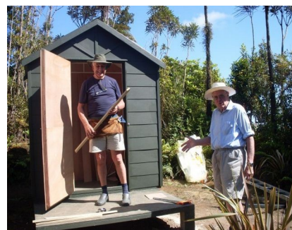
Some of the building team Graeme ZL2TE & Pat ZL2PJ
