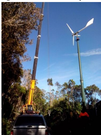
Removing the wind turbine from tower with crane
